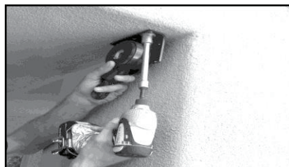
Gear End Bracket
