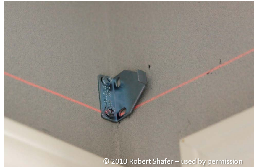
Existing shade bracket with shade removed. Note the line at the level of the lower mounting screw.
