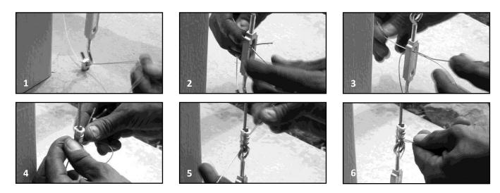
Using left over cable, unravel two strands of wire about 10" in length. Weave strands of wire through tie wire, turnbuckle and then cable loop. Use pliers to twist wire tight. Cut off excess. This prevents the turnbuckle from twisting and loosening the cables. You will repeat this on the other side.
