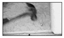
Use Plumb Line to hang from hole in housing (where pointing to in picture) down to ground. Mark spot with pencil for cable anchor. Drill hole with ¼" masonry drill bit. Hammer in tie wire drives. [NOTE: Tie wire drives should be hammered in as far as they can go.] Repeat process on the other side.
