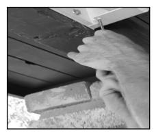
Remove hood screws on both sides of housing located underneath the brackets and set aside.
