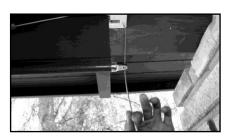
Insert cable through clamp and using a flat head screwdriver, tighten down the setscrew.
