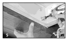
[STEPS 1-3] Once you decide where your housing will hang, hold back of housing up to surface and starting on one side, drill starter holes into mounting surface and secure first lag screw and washer on top hole. Make sure your housing is level. Repeat process on other side of housing.
