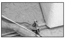
Open turnbuckles by unscrewing each end until ¼" thread remains inside turnbuckle housing. Attach hook end of turnbuckle to tie wire drive.
