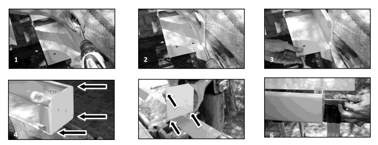
[STEPS 1-3] Start at one end of housing and remove 3 screws attached to housing and set aside. Repeat same process on other side of housing.
