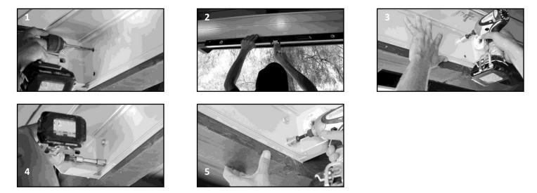
[STEPS 1-3] Once you decide where your housing will hang, hold back of housing up to surface and starting on one side, drill starter holes into mounting surface and secure first lag screw and washer on top hole. Make sure your housing is level. Repeat process on other side of housing.
