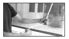
Slide hook end of hand brace into eyelet of gear on shade. Rotate hand brace in one direction to raise. Rotate in opposite direction to lower. Shade rolls up and down on cable guides.
