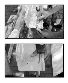
FOR BABY GRANDE: Starting at one at end of housing, make two mounting hole marks 1 1/4" in from end cap on your housing. This is so that the bolt heads will not be behind the fabric roll so they cannot contact the fabric and damage it. You will need to 'toe nail' the bolts (insert at an angle.)
