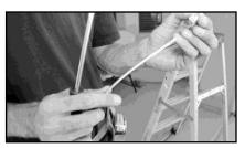
At the top of the cable, you will find a small cable clamp that is already attached. With a flat head screw driver, unscrew front setscrew and remove clamp from cable. Set aside.
