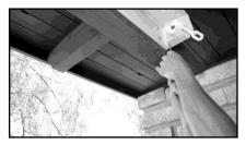
Remove hood screws on both sides of housing located underneath the brackets and set aside.
