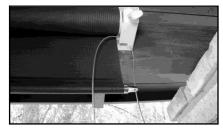
Slip cable up through the eyelet of bottom rail and push up through small hole in bottom of end cap. Continue pulling until top of cable is in reach for you to grasp. Using cable cutters, cut cable to proper length.
