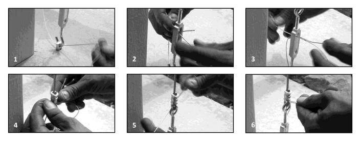
Using left over cable, unravel two strands of wire about 10" in length. Weave strands of wire through tie wire, turnbuckle and then cable loop. Use pliers to twist wire tight. Cut off excess. This prevents the turnbuckle from twisting and loosening the cables. You will repeat this on the other side.
