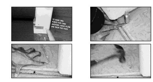
Use Plumb Line to hang from hole in housing (where pointing to in picture) down to ground. Mark spot with pencil for cable anchor. Drill hole with ¼" masonry drill bit. Hammer in tie wire drives.
