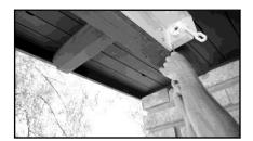
Remove hood screws on both sides of housing located underneath brackets. Set aside.
