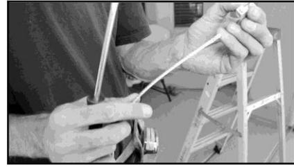
head screw driver, unscrew front setscrew and remove clamp from cable. Set aside.
