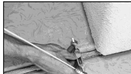
Open turnbuckles by unscrewing each end until  $\frac{1}{4}$ " thread remains inside turnbuckle housing. Attach hook end of turnbuckle to tie wire drive.
