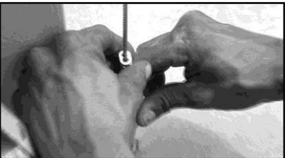
Close turnbuckles to add tension to cables. (Hold top and turn buckle clockwise).
