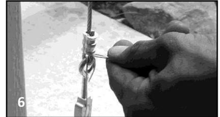
Using left over cable, unravel two strands of wire about 10" in length. Weave strands of wire through tie wire, turnbuckle and then cable loop. Use pliers to twist wire tight. Cut off excess. This prevents the turnbuckle from twisting and loosening the cables. You will repeat this on the other side.
