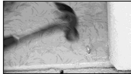
Use Plumb Line to hang from hole in housing (where pointing to in picture) down to ground. Mark spot with pencil for cable anchor. Drill hole with  $\frac{1}{4}$ " masonry drill bit. Hammer in tie wire drives. **[NOTE: Tie wire drives should be hammered in as far as they can go.]** Repeat process on the other side.
