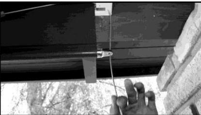
Insert cable through clamp and using a flat head screwdriver, tighten down the setscrew.
