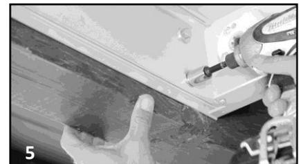
[STEPS 1-3] Once you decide where your housing will hang, hold back of housing up to surface and starting on one side, drill starter holes into mounting surface and secure first lag screw and washer on top hole. Make sure your housing is level. Repeat process on other side of housing.
