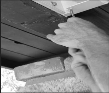
Remove hood screws on both sides of housing located underneath brackets. Set aside.
