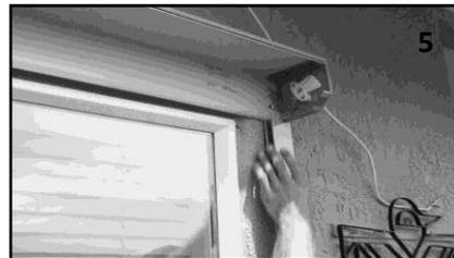
FOR OUTSIDE MOUNT, starting on one side, place side rail on flat surface directly underneath housing, making sure it is flush (#1).
