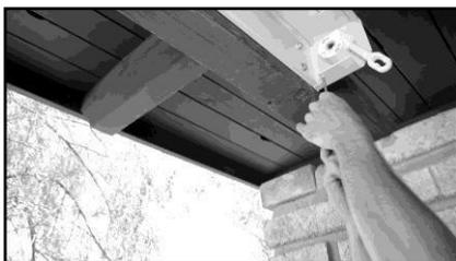
Remove hood screws on both sides of housing located underneath brackets. Set aside.
