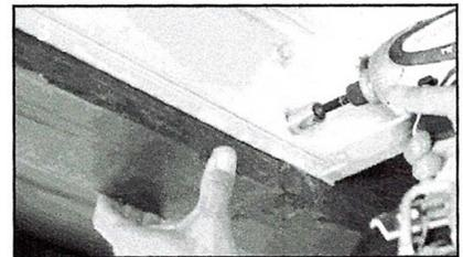
Once you decide where your housing will hang, hold back of housing up to surface and starting on one side, drill starter holes into mounting surface and secure first lag screw and washer on top hole. Make sure your housing is level. Repeat process on other side of housing.
