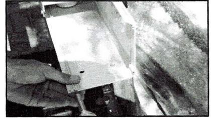
Start at one end of housing and remove 3 screws attached to housing and set aside. Repeat same process on other side of housing. **Slide shade brackets into channel on back of housing and tap in gently with a hammer.** Once brackets are in place attach end caps to back of housing.
