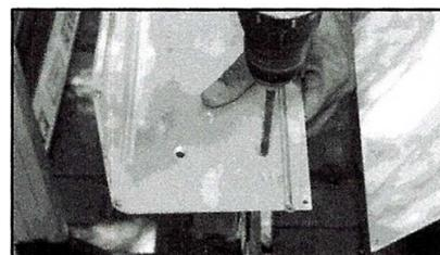
Starting at one at end of housing, make two mounting hole marks 1 1/4" in from end cap on your housing. Using a 3/8" metal drill bit, drill the two mounting holes. Repeat this process on other side of housing with other end cap.
