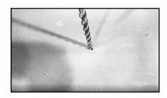
Drill hole with ¼" masonry drill bit.
