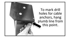
Use Plumb Line to hang from hole in housing (where pointing to in picture) down to ground. Mark spot with pencil for cable anchor.
