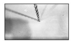
Drill hole with ¼" masonry drill bit. Hammer in tie wire drives.
