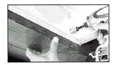
Once you decide where your housing will hang, hold back of housing up to surface and starting on one side, drill starter holes into mounting surface and secure first lag screw and washer on top hole. Make sure your housing is level. Repeat process on other side of housing.
