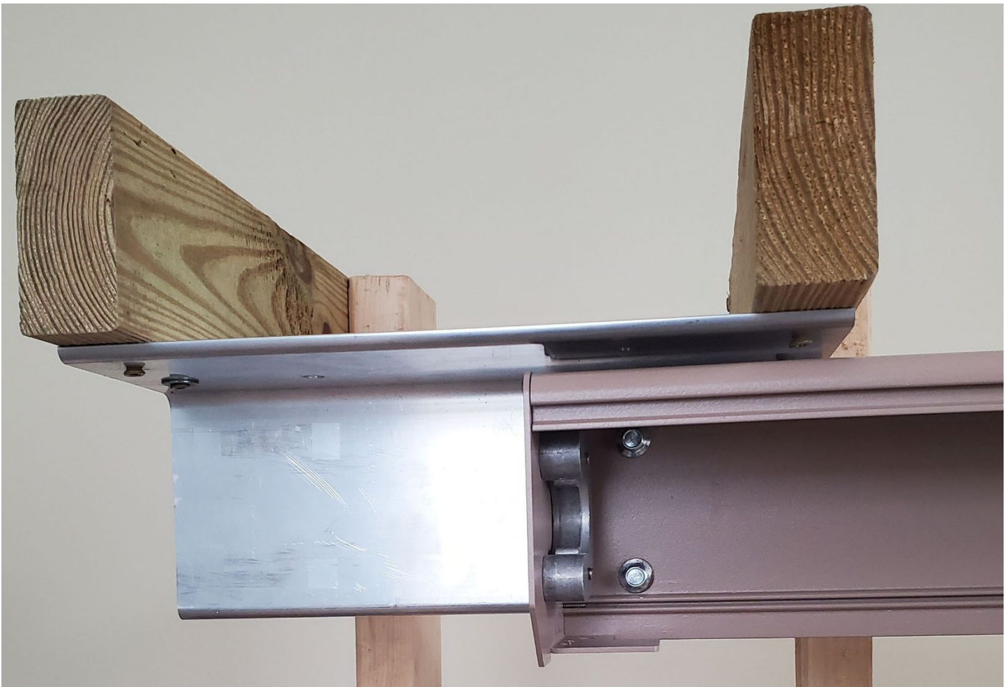
Under mounting to rafters (where mounting fasteners do not line up with a rafter)
