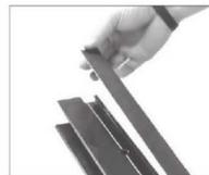
e. From the full length of the cut side track, remove snap-in track cover.
