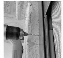
e. Install the track cover working from top to bottom.
